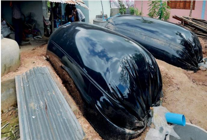
The biogas system in the household uses ten sacks (600 kilograms) of pig manure to be fermented in a cement pond that is dug into a 1-meter deep hole, 1.5 meters wide and 4 meters long, with PE sheet covering. A cement pond for pig manure, food waste should be filled one time a day. The system from the gas wells will be connected to the burner. A stove for households will receive 2-3 cubic meters of gas
